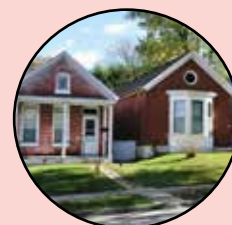
TRAPP ROW, C. 1889 Small houses referred to as "Shotgun cottages" built on 30-ft lots in Calftown 303-321 S 10TH
